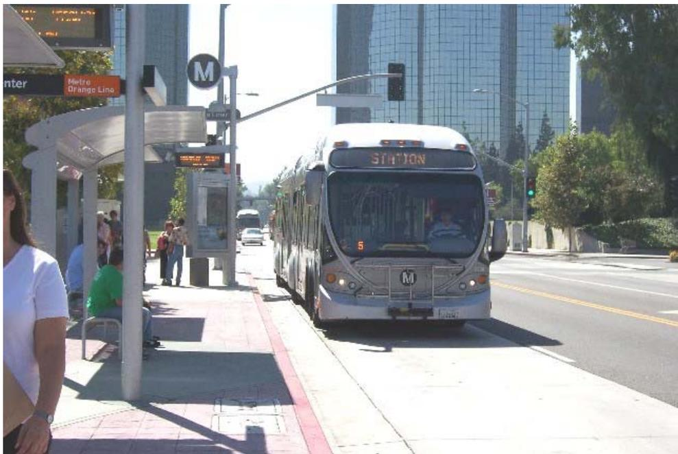
**Figure 2. Mixed traffic lane in an urban setting with no parking and a view of the curb (Orange Line, Los Angeles).**
