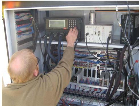
Figure 4.10 Program Eagle Traffic Signal Controller
