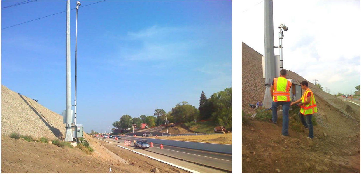
Figure 7. HWY 280 work-zone site deployment of portable traffic video data collection apparatus.
