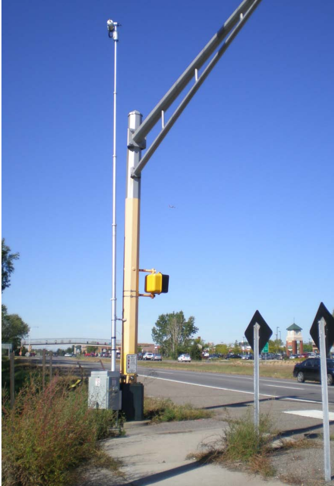
Figure 5. Camera location with respect to chosen stop bar line at HWY 55 & Rhode Island Ave. intersection.
