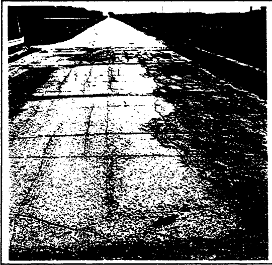
Figure 4 - Longitudinal and Transverse Pavement Cracking on a Field Laminated LNL Deck
