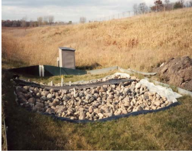
Figure 1.2. Completed Check Dam August 2001.
