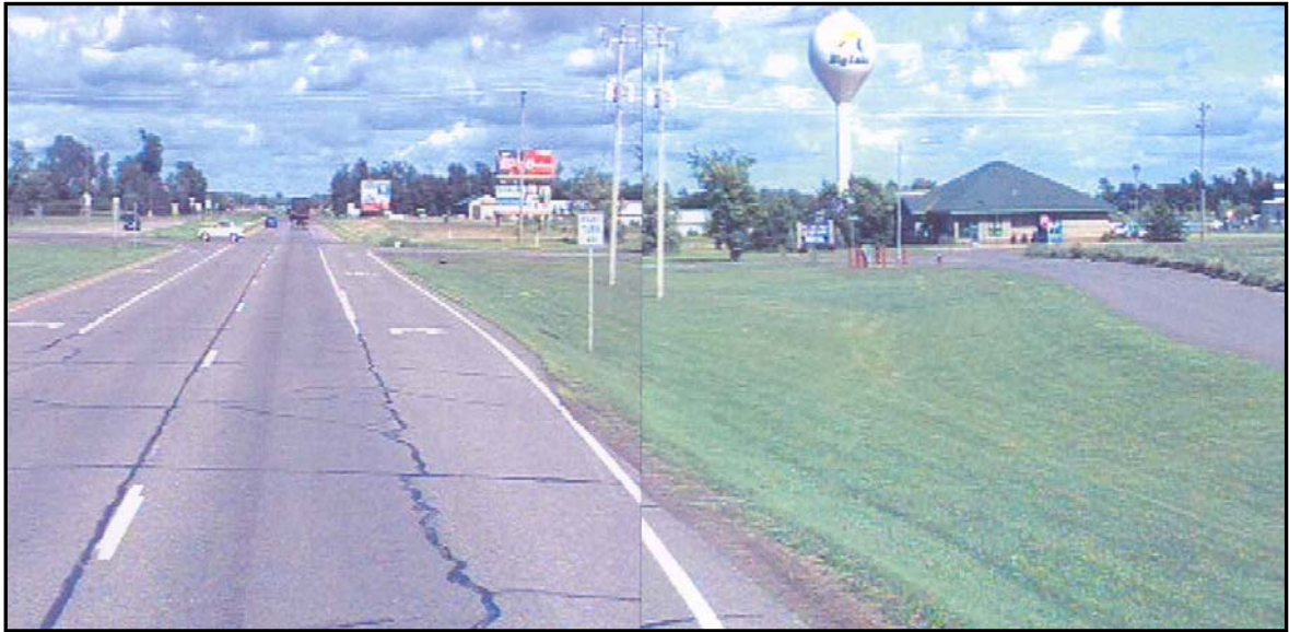
Figure A-4: Eastbound US 10 at CR 43 (Big Lake)
