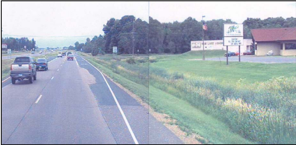
Figure A-5: Northbound MN 65 at 177th Avenue (Ham Lake)
