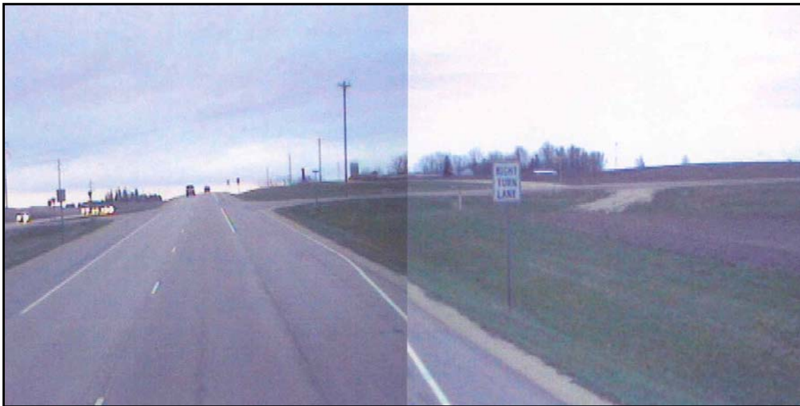
Figure A-2: Southbound US 52 at CSAH 9 (Goodhue County)
