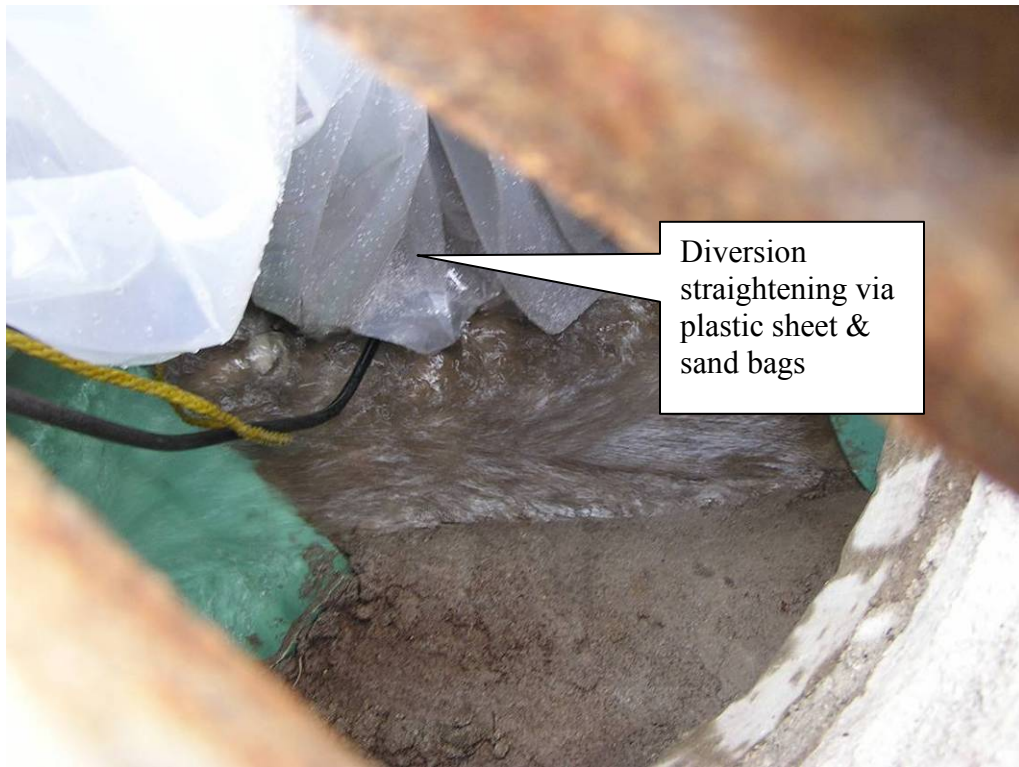
Figure C.6: Use of a plastic sheet weighed down with sandbags to smoothly turn water downstream toward the V2B1 (water moving right to left) and therefore eliminate coarse sand particle settling in front of the inflatable plug due to weak vortices.
