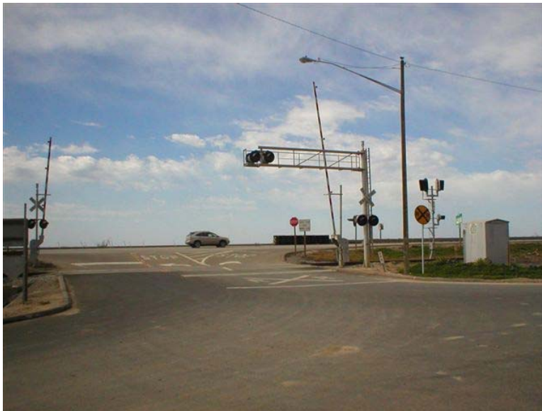
FIGURE 4-3 La Conchita Road Approach
