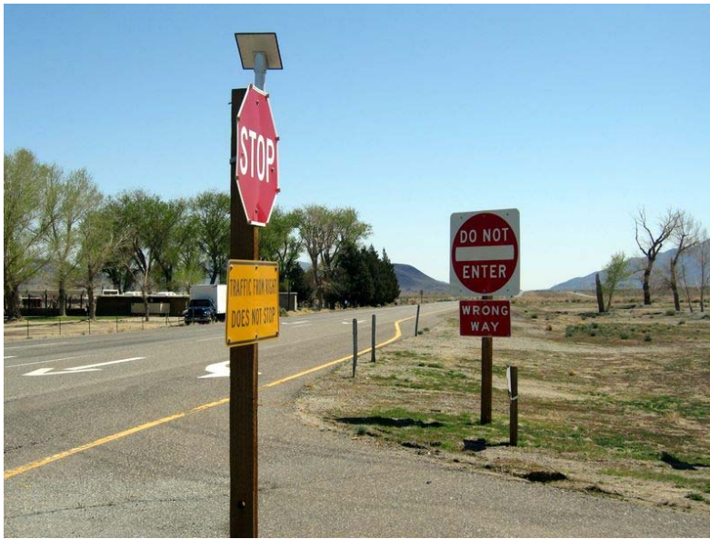
FIGURE 4-6 Sight Obstruction While Looking South from the Median
