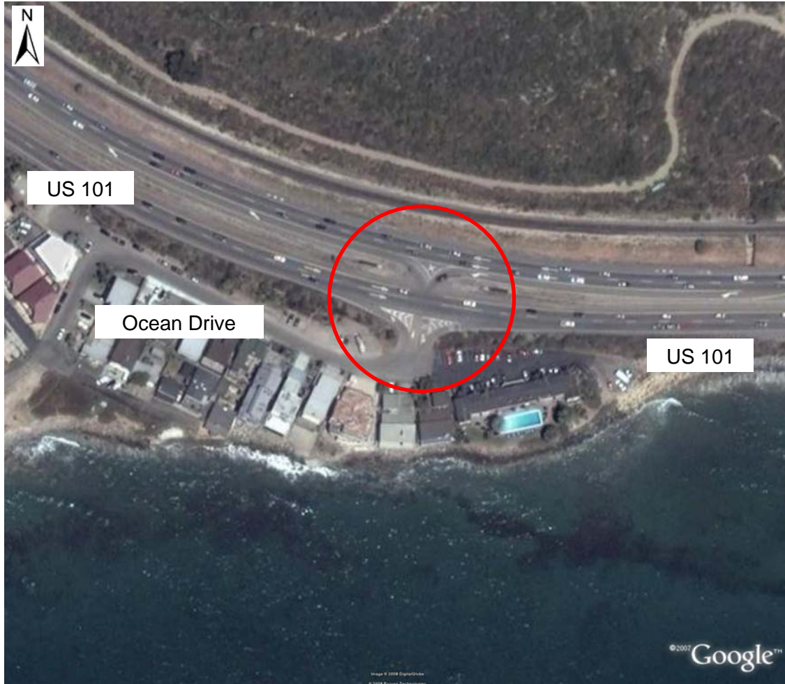
FIGURE B-1 Aerial Photo of US 101 & Ocean Drive (Ventura County)
