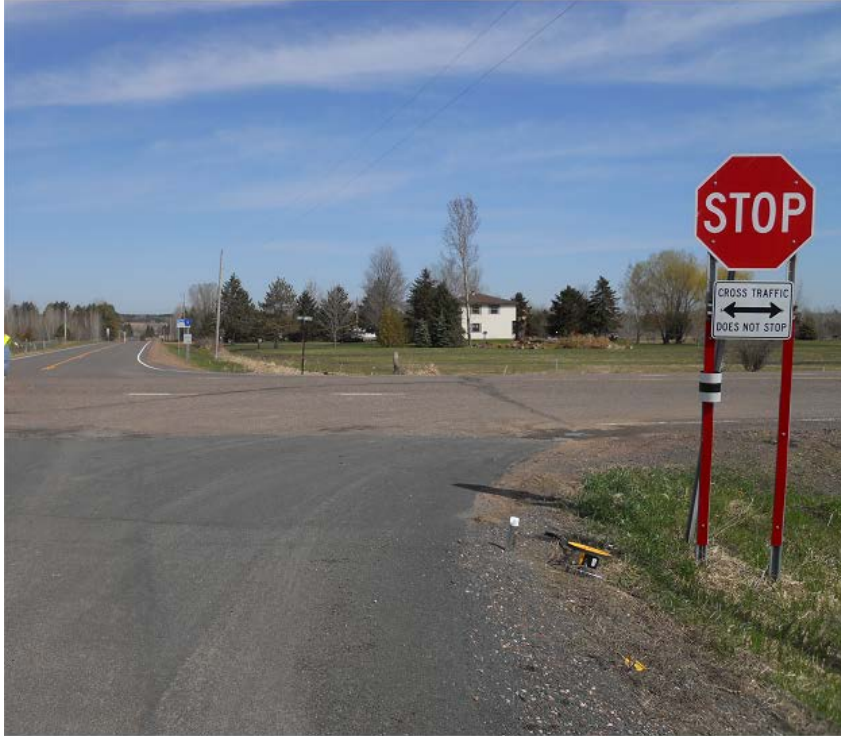
Figure 3.5 Anchoring Post and View Looking North at MNTH 95 and Chisago CSAH 9
